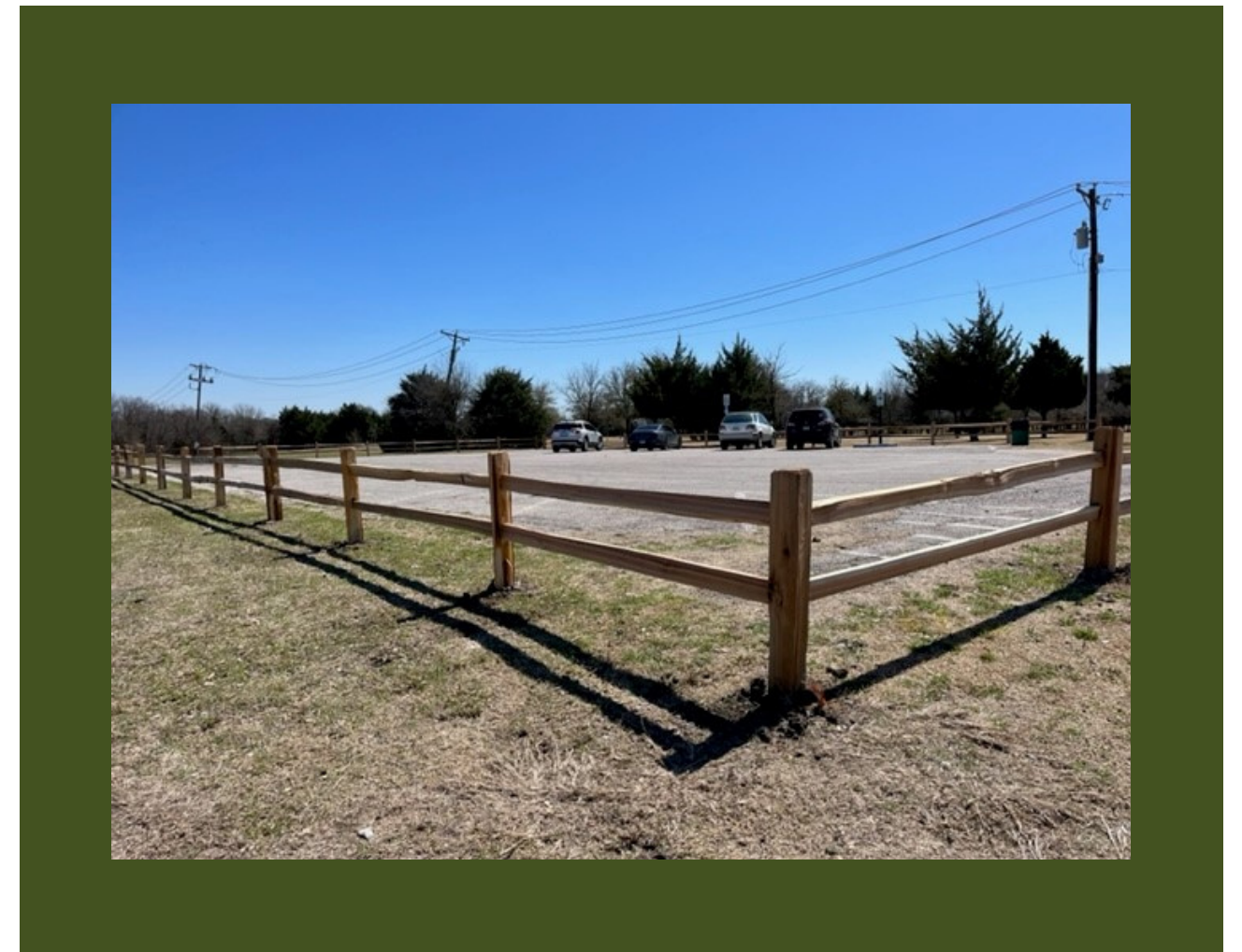
FOXCHASE PARK SPLIT RAIL FENCE INSTALLATION
